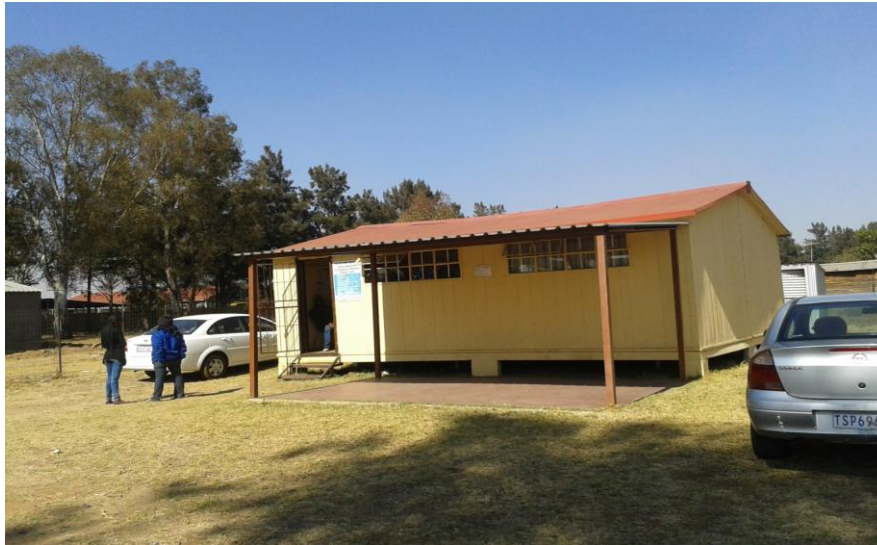
Fig 3: A health post in Boipatong ward in Emfuleni sub-district
